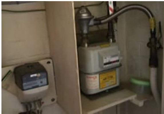
Asbestos panelling around a gas meter
